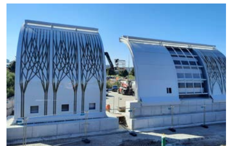
For the snow breakaway edge each angle had to be computed and manufactured individually.
